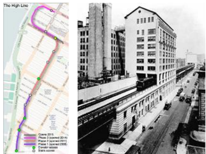
Fig. 6. Unused Rail Structure in 1936 and Context
