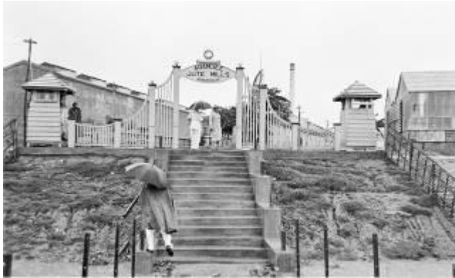
Fig. 1. Entry in Adamjee from Shitalakkha River, 1964
