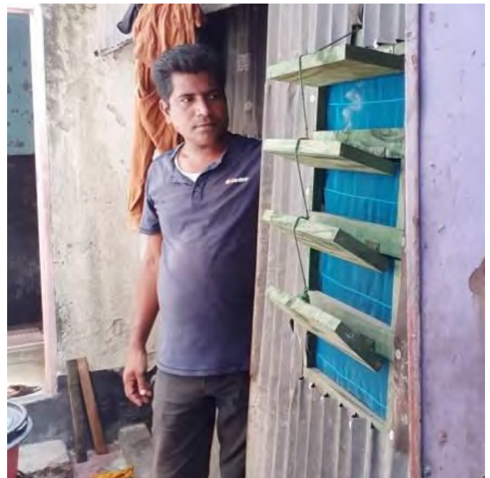
Fig 17: Designed window modules with operable louvered panels and fixed mosquito net have been retrofitted in the existing façade to improve ventilation condition
