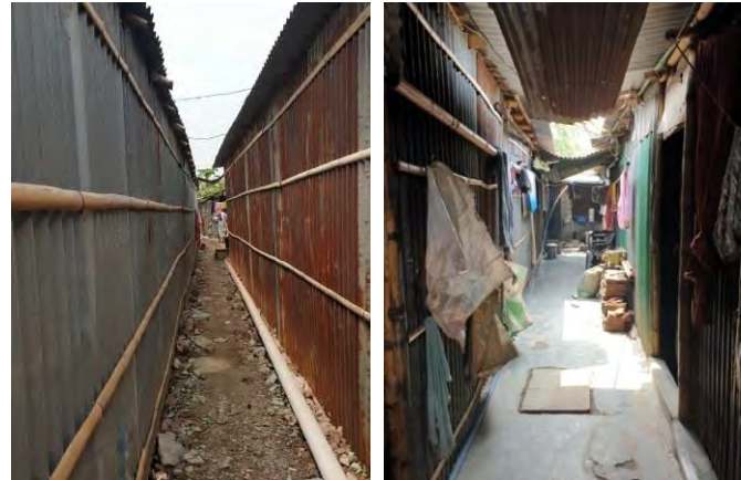
Fig 06: Dwelling units without any openings, because of narrow setback and access way
