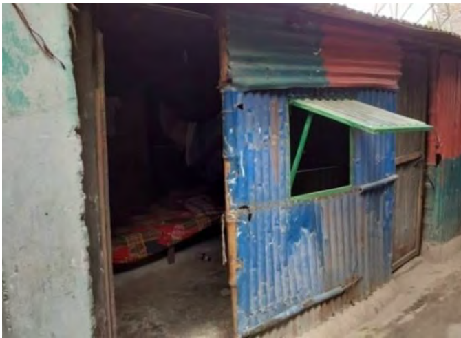
Fig 18: Designed window modules with fixed semi-transparent polycarbonate sheet in wooden frame have been retrofitted in the existing façade to improve Day light. Before this retrofitting, these units were completely dark during daytime.
