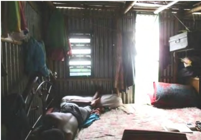
Fig 19: Designed window modules with fixed semi-transparent polycarbonate sheet and louvered panels have been retrofitted in the existing façade to improve Day light and Ventilation condition. Before this retrofitting, these units were completely dark during daytime, and had no option for ventilation.
